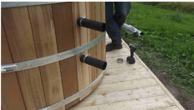
*Fig. 10.2.2 Attach heater hoses with gear clamps*
