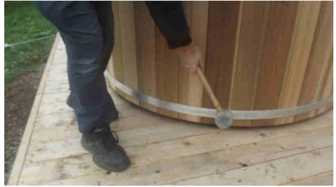
Figure 9.1 Hitting staves directly on the strap.
