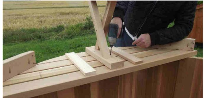
Fig. 10.1.2 Attach bench brackets with supplied 2" screws.
