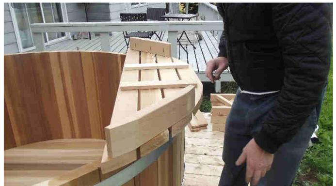
Fig. 10.1.3 Bench Brackets Flush with ends of benches,  $\frac{3}{4}$ " from wall.
