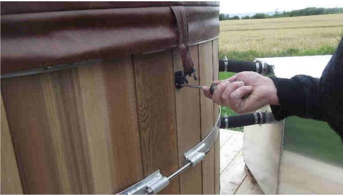
Fig. 10.4.1 Attaching the cover strap buckle.
