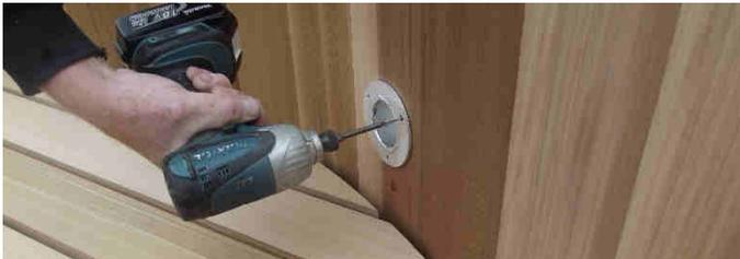
*Fig. 10.2.1 Fasten heater hose fitting.*
